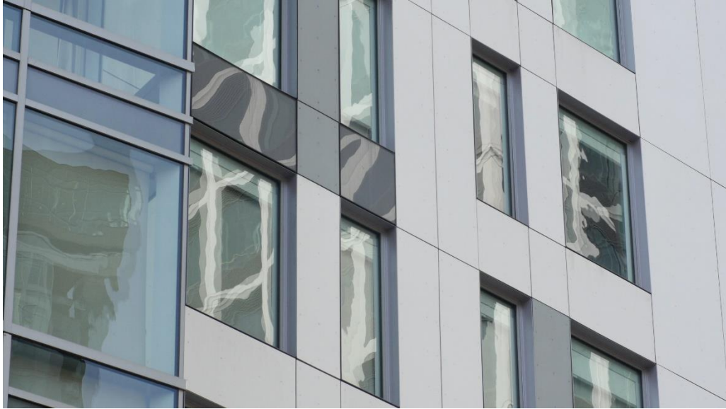
Figure 4. Architectural panels bonded with acrylic foam tape
