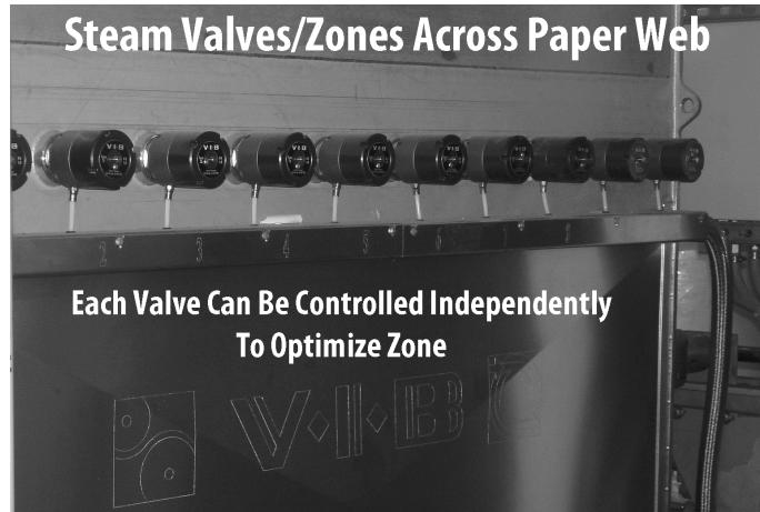
Figure IV: Steam Valves and Zones in Re-Moisturizer
