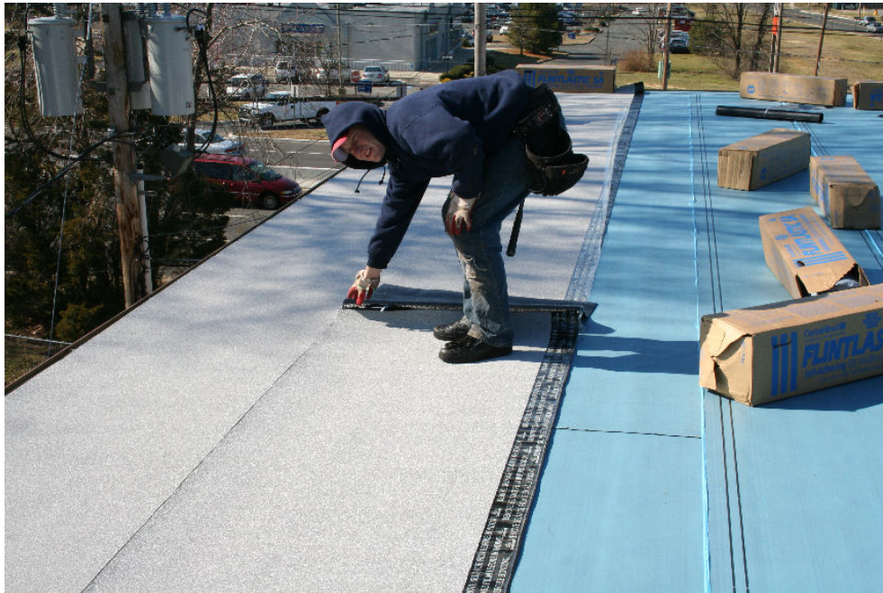
Figure 6, granulated self adhered cap sheet over film topped ply sheet
