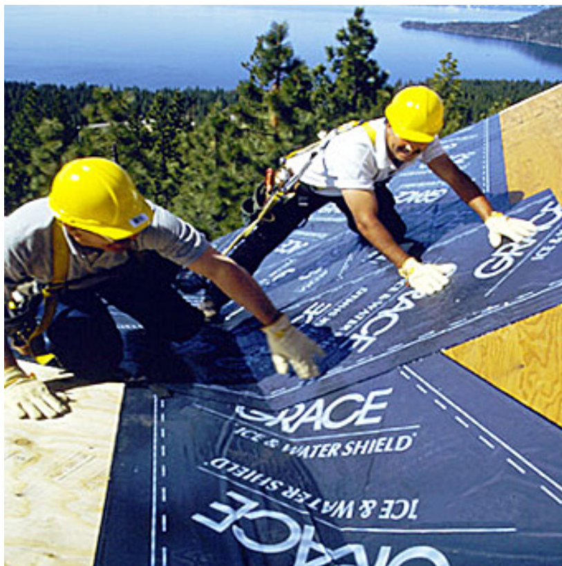
Figure 4, ice and water dam protection
